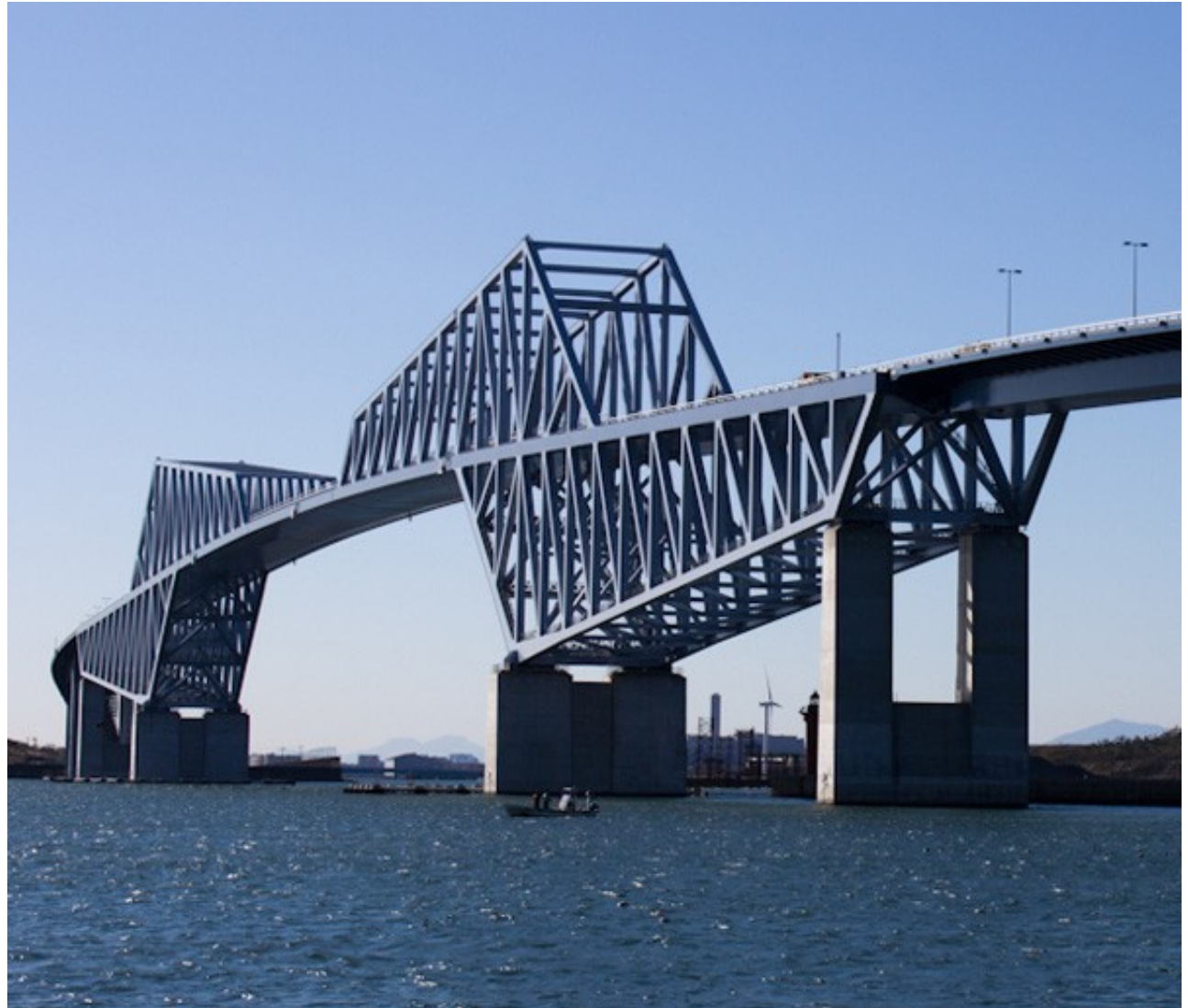
Tokyo Gate Bridge , a 2.6km long truss bridge
